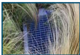
Above photos show rock pile, overgrown weeds, and flower bed blocking roadside swale inlets.
